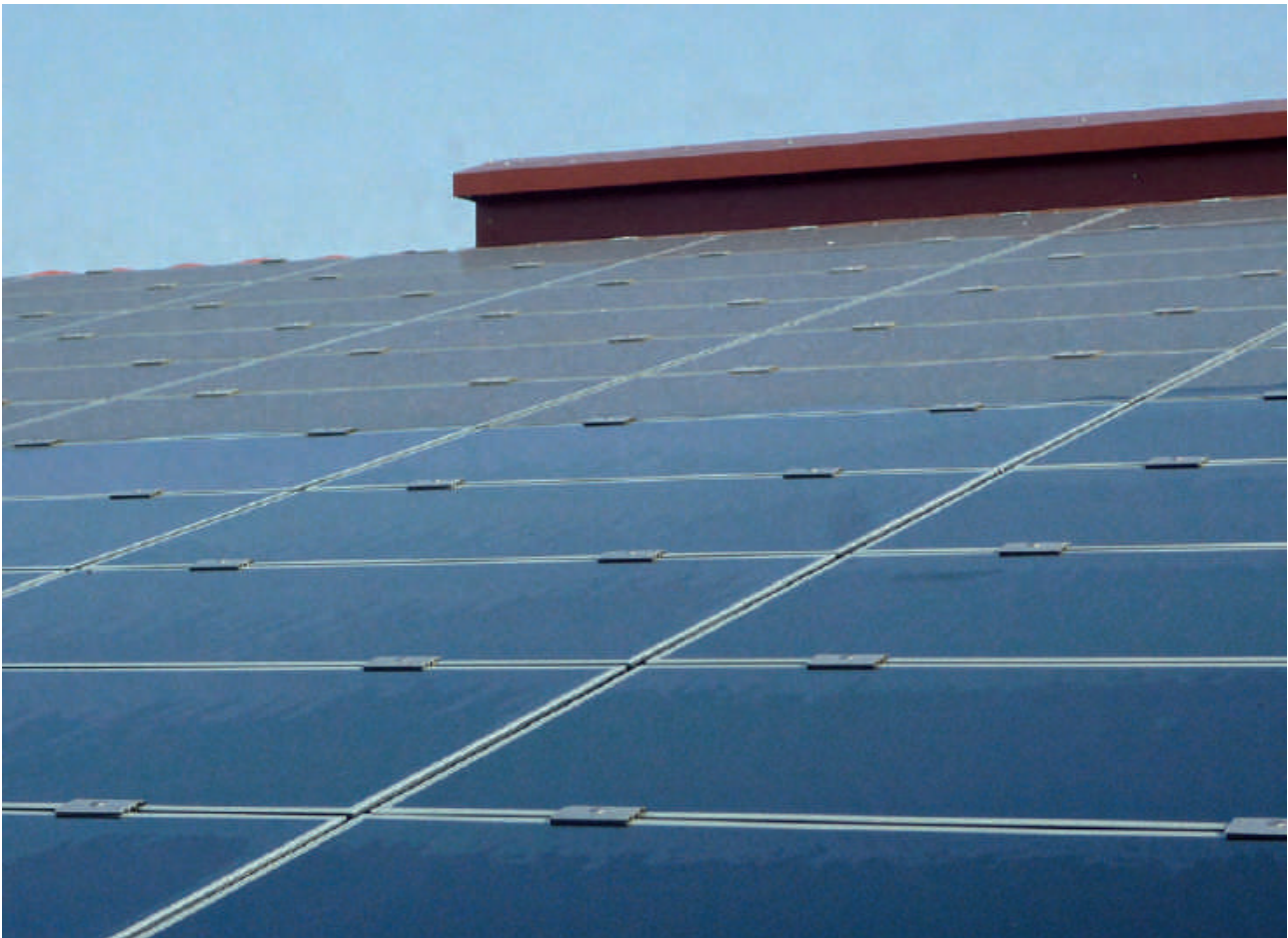
Image 6: Comparison between cleaned modules (lower rows) and uncleaned modules (upper rows) at Farm 2
