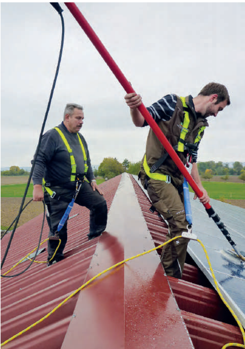
Image 8: Two people on roof cleaning downwards.
